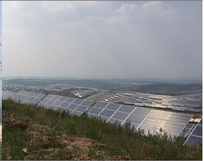
Figure 6: UPV’s Datong project
